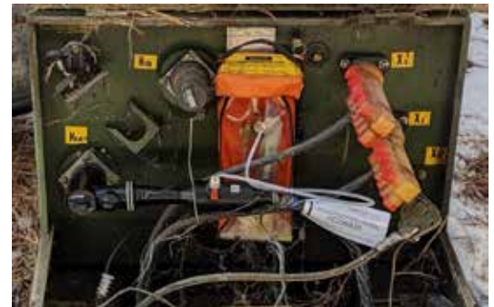
Figure 2: MIC Injection in a low-profile transformer
