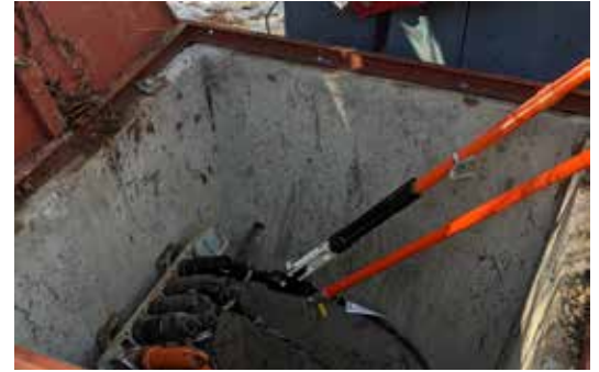
Figure 3: Completing MIC injection in a vault
