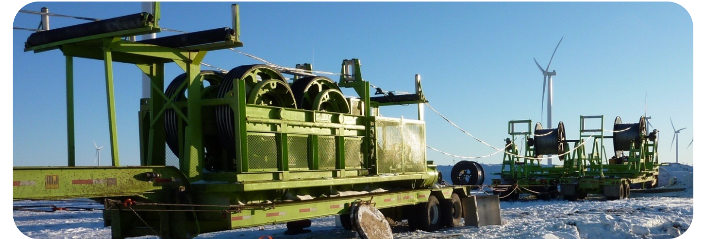
Figure 8: Payoff and bullwheel setup.
