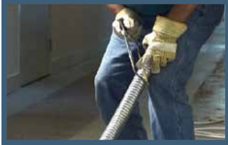
Using hacksaw to cut two adjacent convolutions
