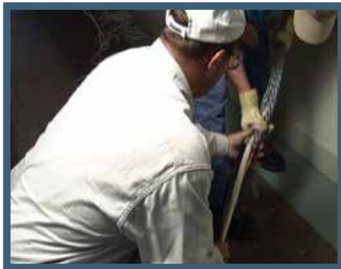
Securing pull rope to cable assembly
