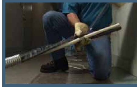
Removing mylar tape from conductors
