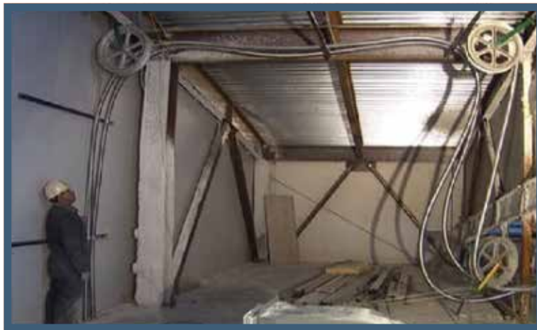
Example of using multiple sheave wheels to achieve required bending radius
