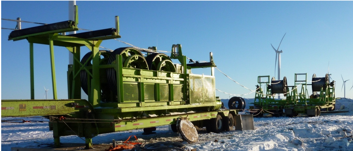
Figure 5. Payoff and bullwheel setup.
