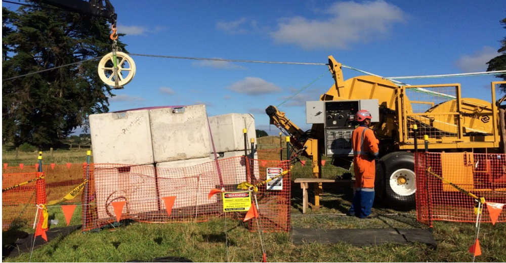
Figure 9. Suitable technique for roller diversion, courtesy of Transpower New Zealand.
