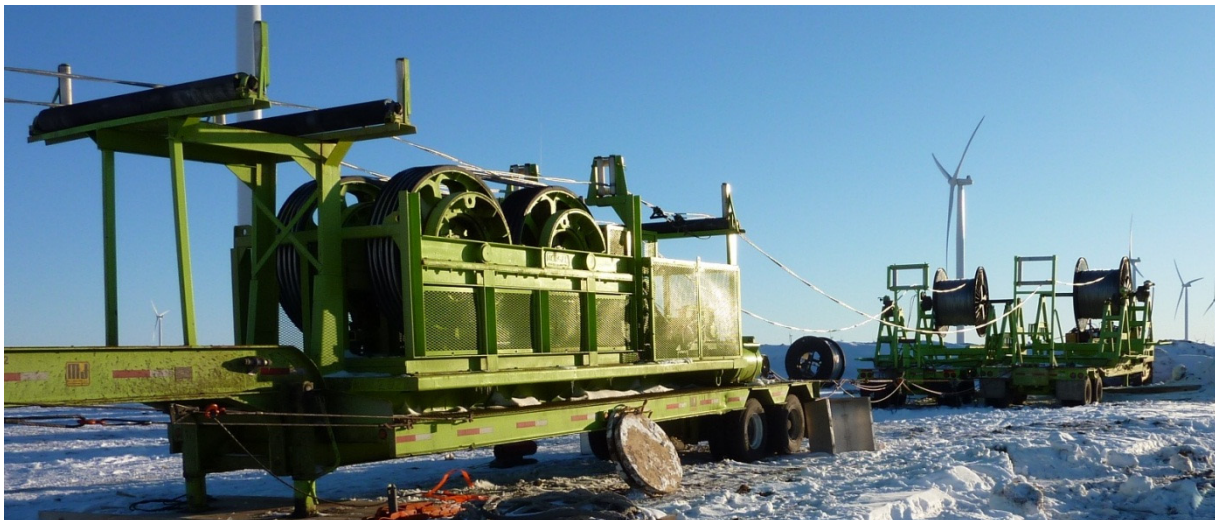
Figure 6. Payoff and bullwheel setup.
